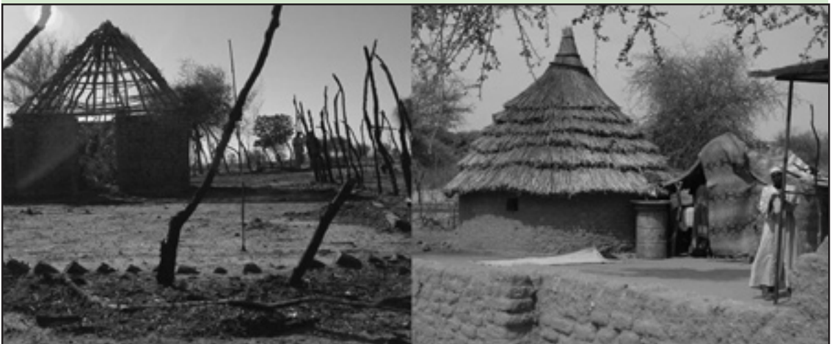
Destroyed and Rebuilt Village, Sudan. Photo: Michael Wadleigh
